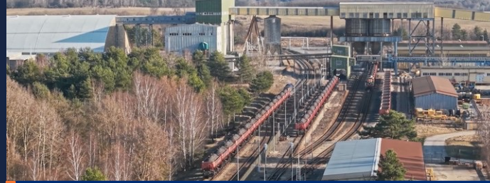
Rail loading yard at the smelter
